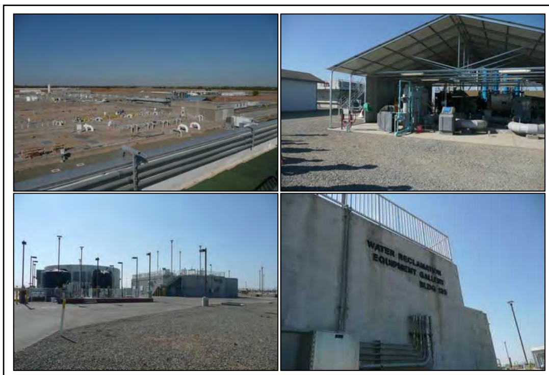
Figure 3.1-2: Existing Facilities at SRWTP
