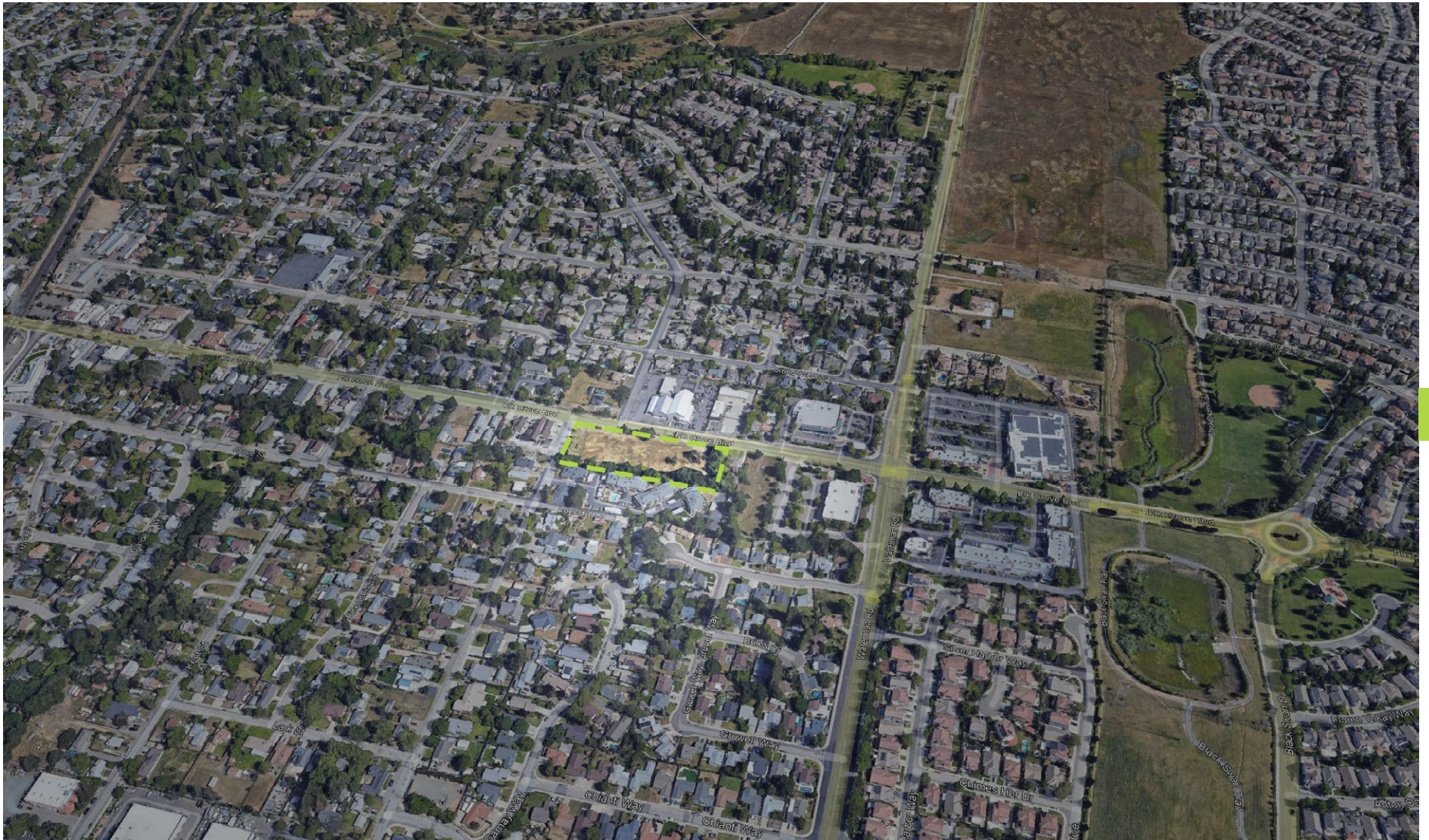
Figure 3. Old Town Site and Surrounding Neighborhood, Looking North
