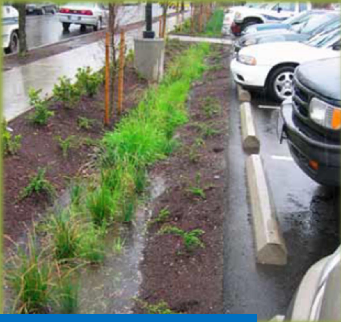
Bioretention and grassy swale
