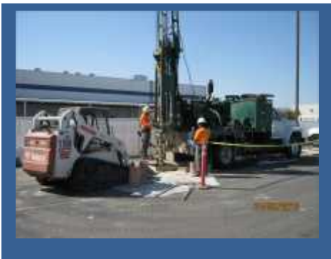
Drilling Monitoring Wells
