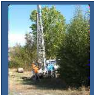
Strawberry Creek Water Quality Basin – Drilling Dry Well
