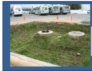
Corporation Yard – Sedimentation Basin, Dry Well and Bioswale Construction
