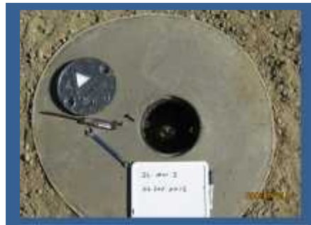
Completed Downgradient Well (MW3)
