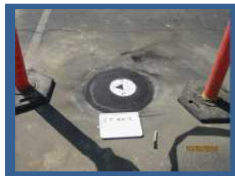
Completed Downgradient Well (MW4)
