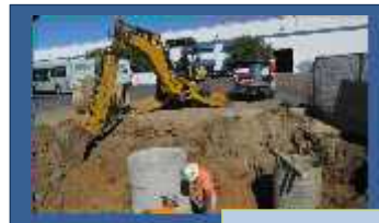
Corporation Yard – Sedimentation Basin, Dry Well and Bioswale Construction
