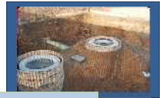
Corporation Yard – Sedimentation Basin, Dry Well and Bioswale Construction
