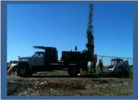
Drilling Monitoring Wells
