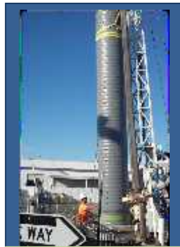
Corporation Yard – Dry Well Casing Installation
