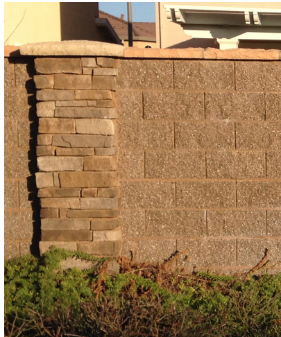
Community Pilaster & Wall
