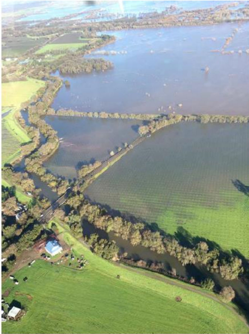
Figure 4-86 New Hope Levee Break
