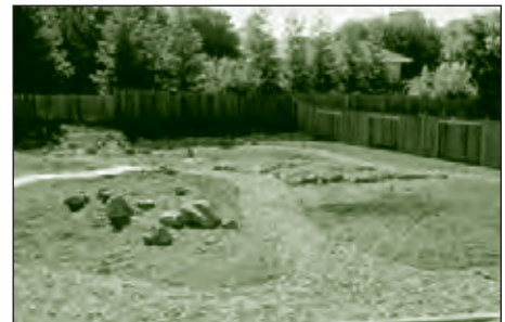
Sheet mulched site is ready for planting.
