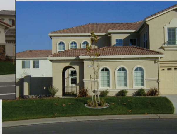
Photo III-73: Third car garage is perpendicular to street with window articulation and announcement of entry
