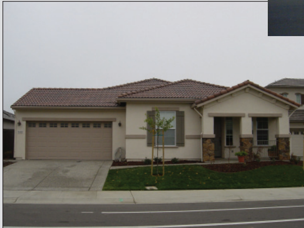
Photo III-74: The darker contrasting color of the garage door minimizes the visual impact of the door from the street
