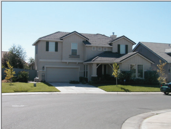
Photo III-40: The home on the left utilizes low second floor exterior wall heights and limits two story design elements
