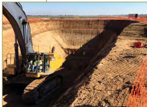
New Growth Area Infrastructure Project 2018
