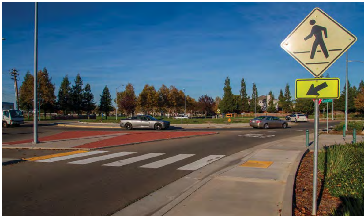
Traffic Circle in East Elk Grove
