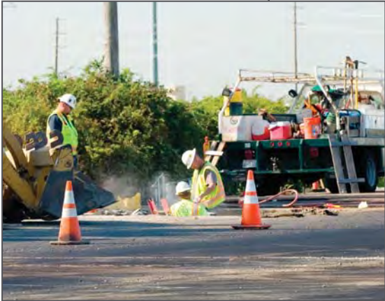
Roadway Construction in Elk Grove
