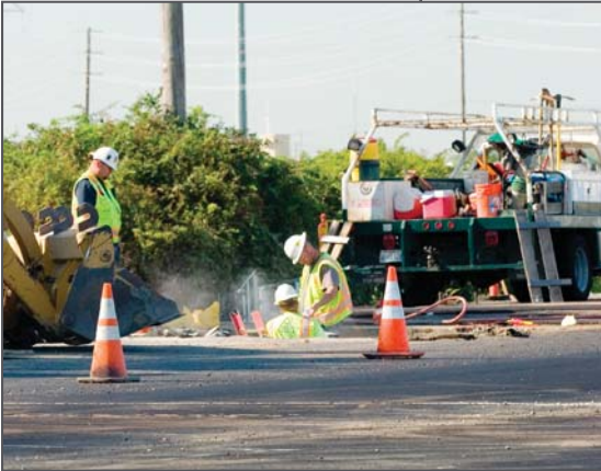
Roadway Construction in Elk Grove
