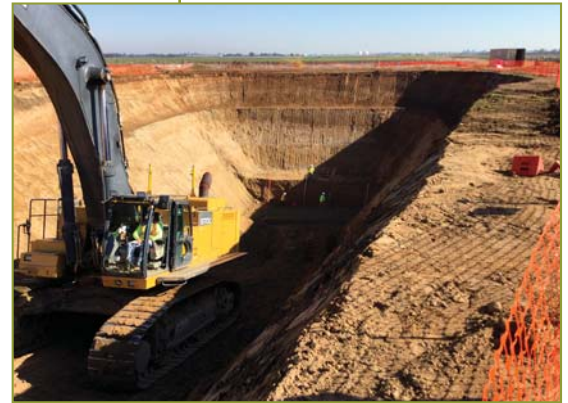
New Growth Area Infrastructure Project 2018
