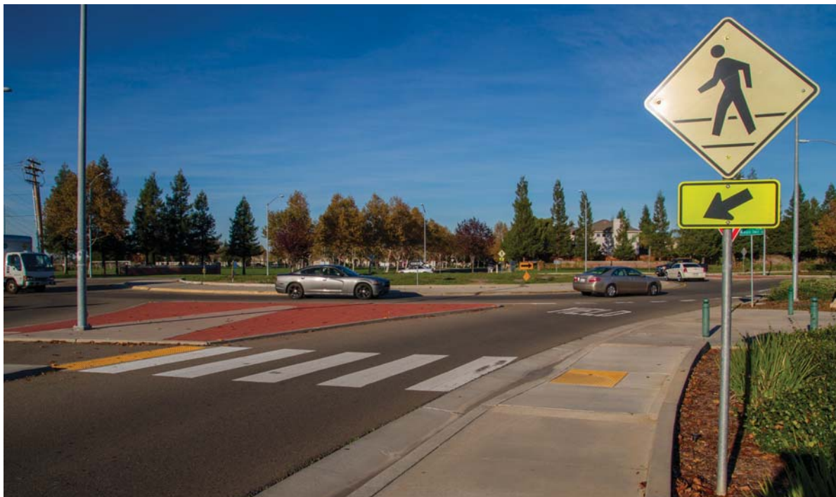
Traffic Circle in East Elk Grove
