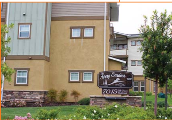
Avery Gardens Apartment Complex in Elk Grove
