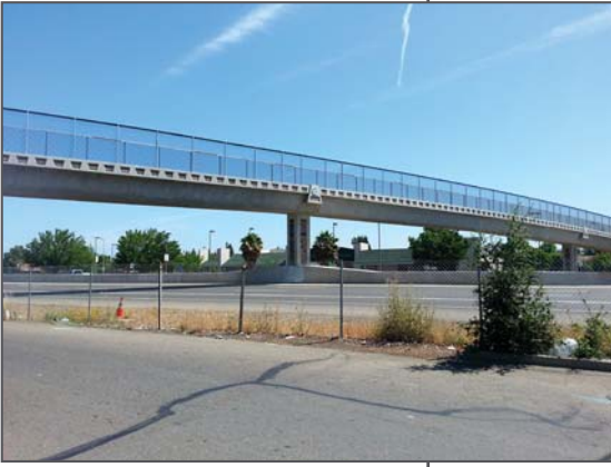
Pedestrian Bridge over SR-99
