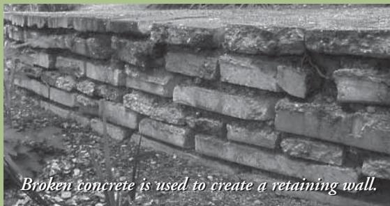
*Broken concrete is used to create a retaining wall.*
