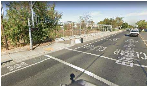
Figure 36. A photo taken from Google Maps Street View from 2020 showing the narrow space just outside of the caged sidewalk forcing bicyclists to make a sharp left turn to cross or wait for the pedestrian signal.
