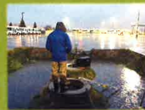
City of Elk Grove Corporation Yard dry well system
