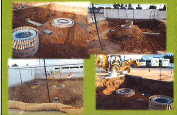
Construction – Corporation Yard
