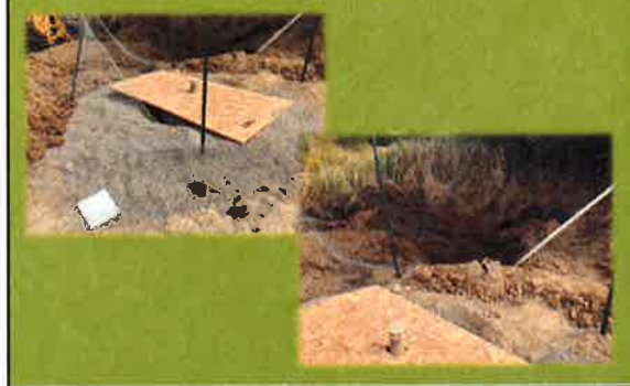
Construction – Strawberry Creek Water Quality Basin
