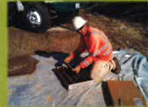
Logging Boring Samples
