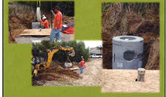
Construction – Strawberry Creek Water Quality Basin
