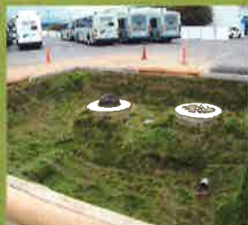
City of Elk Grove Corporation Yard dry well system
