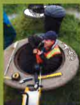
Measuring infiltration rates at the Corporation Yard April, 2015
