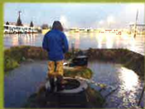
City of Elk Grove Corporation Yard dry well system
