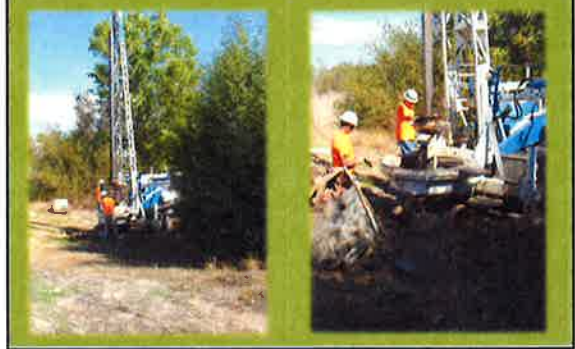
Construction – Strawberry Creek Water Quality Basin
