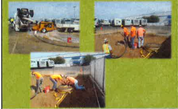
Construction – Corporation Yard
