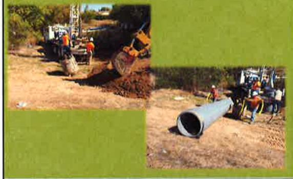
Construction – Strawberry Creek Water Quality Basin
