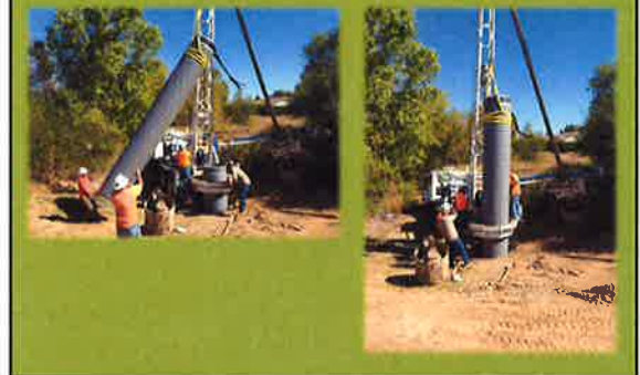
Construction – Strawberry Creek Water Quality Basin
