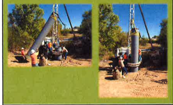
Construction – Strawberry Creek Water Quality Basin
