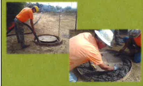
Construction – Strawberry Creek Water Quality Basin
