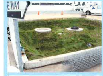
Fig. 1 (above) Grassy swale pretreatment feature at CY site Fig. 2 (below) Installation of perforated drywell casing at CY site
