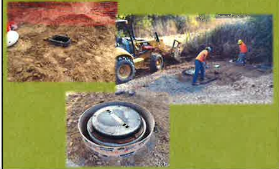
Construction – Strawberry Creek Water Quality Basin
