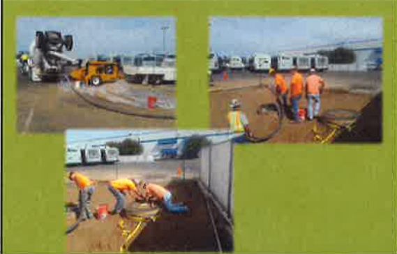
Construction – Corporation Yard
