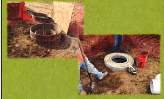
Construction – Strawberry Creek Water Quality Basin
