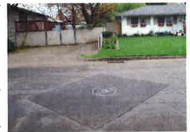
Figure 1. A UIC located in a public right of way. Source: Oregon DEQ UIC program.
