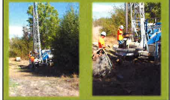
Construction – Strawberry Creek Water Quality Basin
