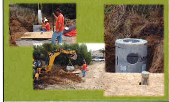
Construction – Strawberry Creek Water Quality Basin
