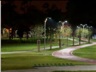
Pedestrian- scaled lighting
