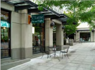
Clearly marked entrances
