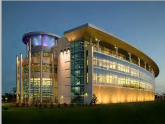
Accent lighting of buildings
