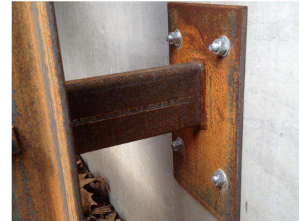
Example of Metal Grid Panel Mounting Bracket, when applicable (Metal Frame to Pilaster)
