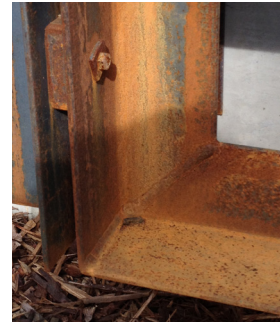
Example of L Channel Outer Frame at corner
