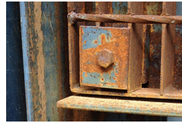
Example of Hex Bolt Attachment/Accent (Metal Grid Panel to Frame)
