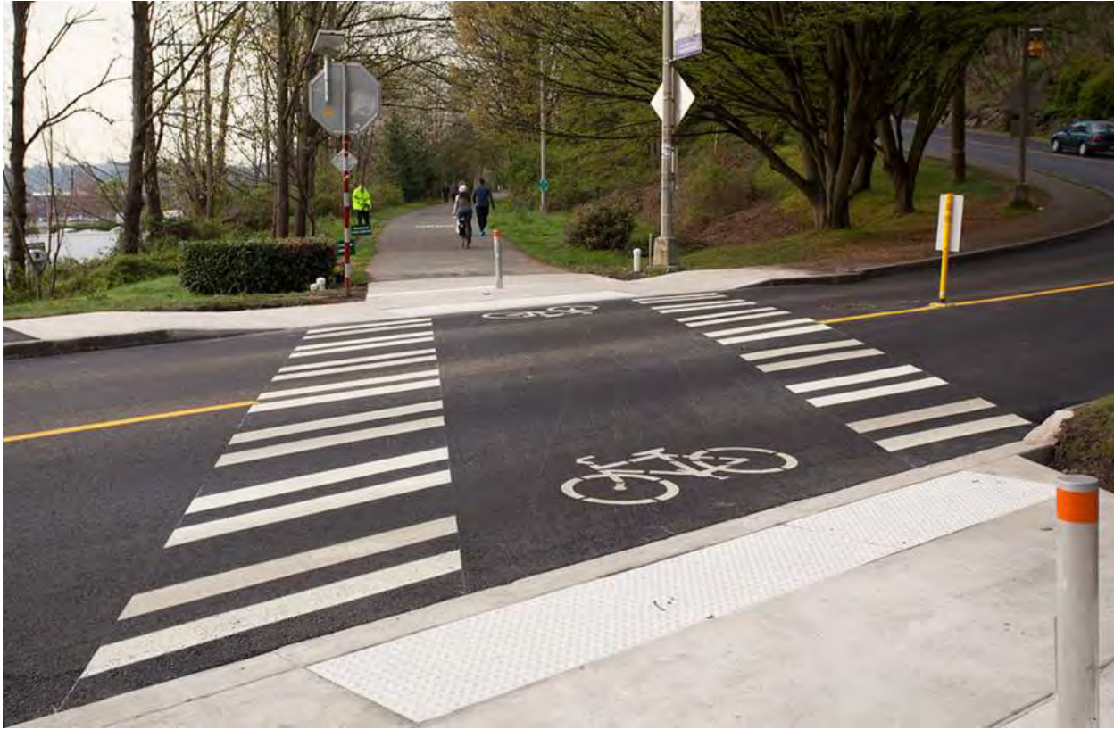
Figure 10. Example of Multi-use Trail Crossing Treatments (a midblock trail crossing is shown).
