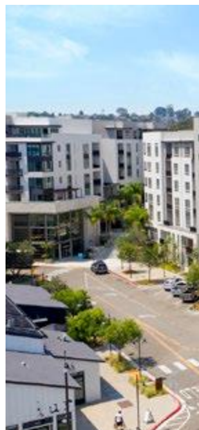
ONE PASEO, SAN DIEGO, TCA ARCHITECTS & GENSLER
