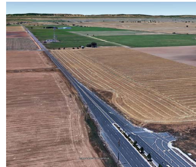
Existing Kammerer Road looking West
