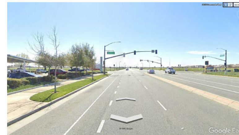
Existing Streetscape - three vehicular lanes in each direction separated by a landscaped center median
