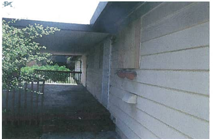
Photo 30 – APN-014 rear of north house
