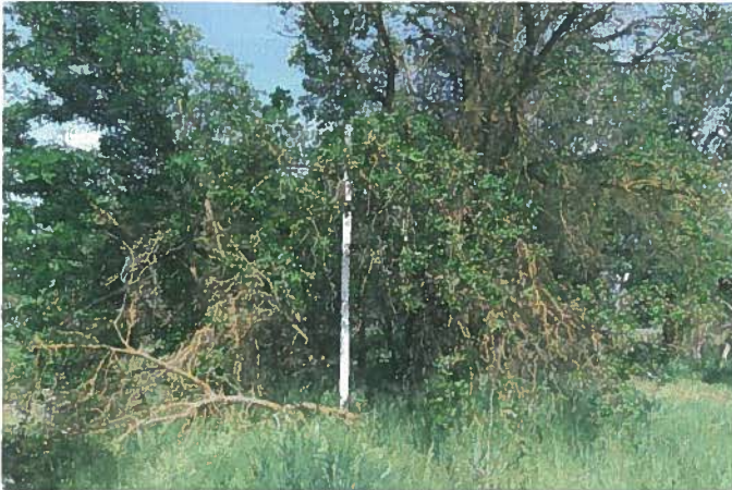
Photo 7 – APN-015 PVC pipe at northwest corner
