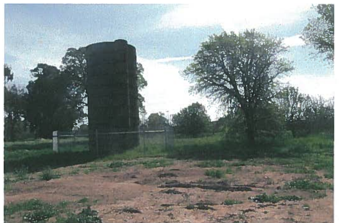
Photo 4 – APN -015 water tower
