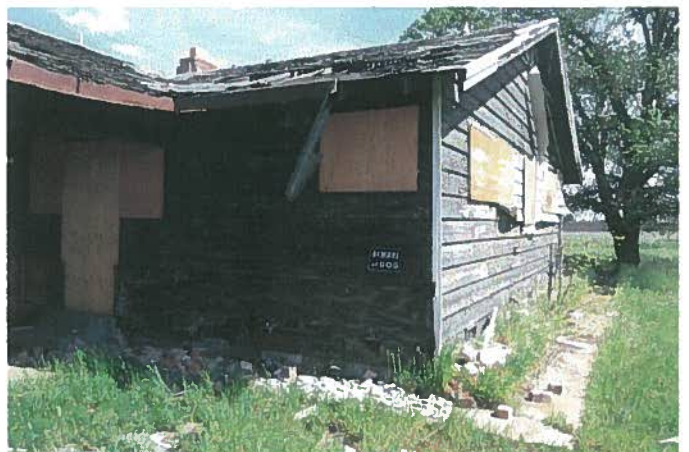
Photo 24 – APN – 014 middle house
