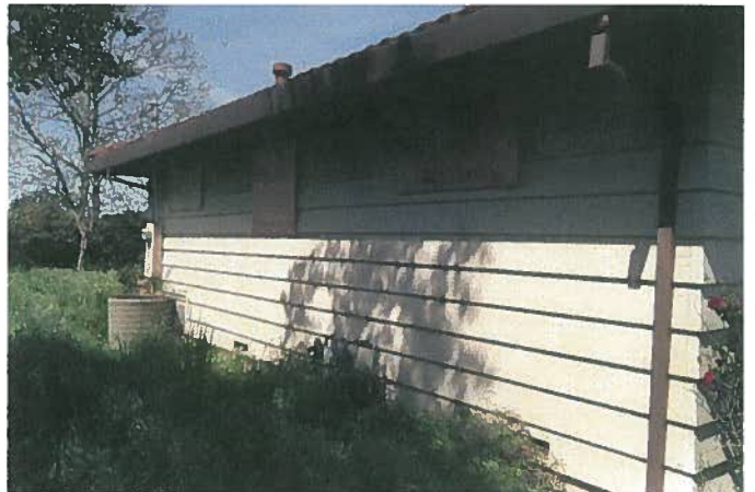
Photo 28 – APN-014 side of north house
