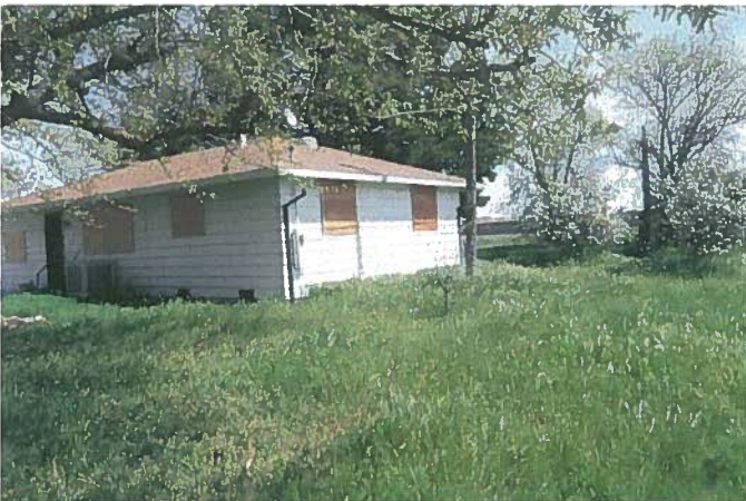
Photo 21 – APN – 014 south house
