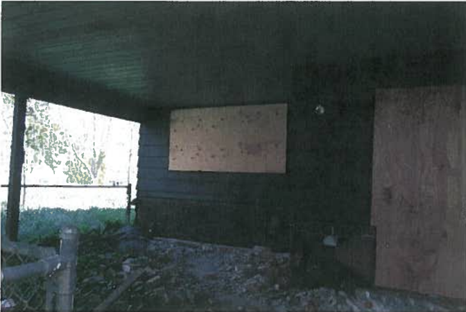
Photo 25 – APN – 014 middle house front
