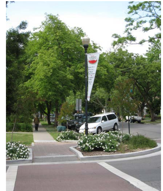
Bulbout at pedestrian crossing
