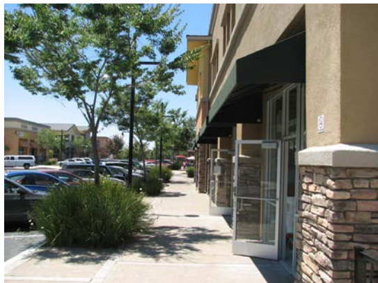
Landscaped buffer and curbside parking between pedestrian and vehicle zones
