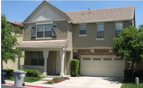
Garage with architectural details – windows
