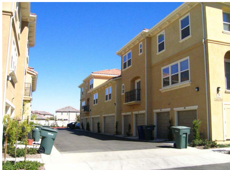
Residential alley and service area
