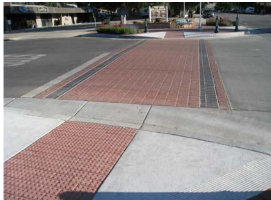
Crosswalk with decorative paving
