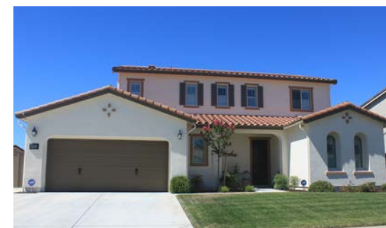
Garage width less than 50% of building width
