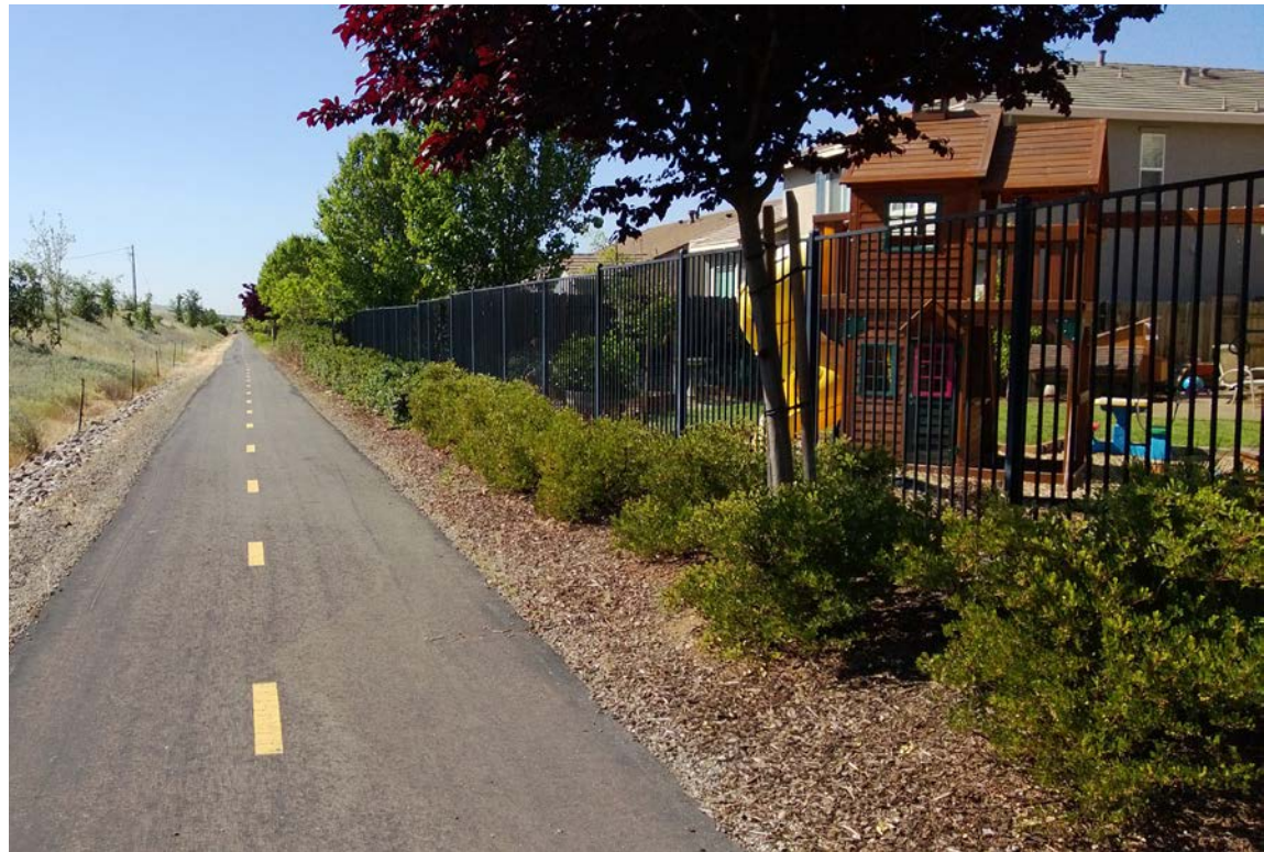
Tubular steel fencing
