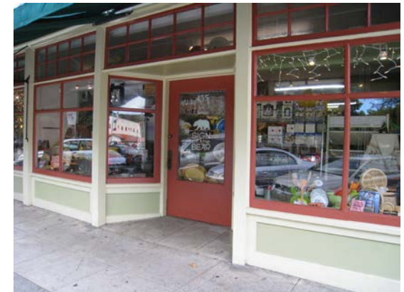
Transparent glass with views into the building
