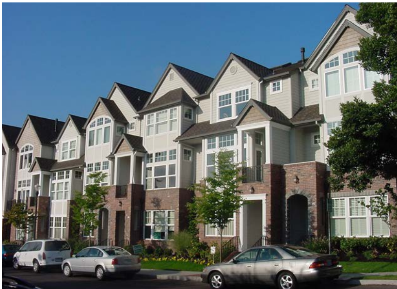
Multiple building materials used on primary façade
