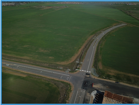
Site Location - NE Corner of Bilby and Big Horn
