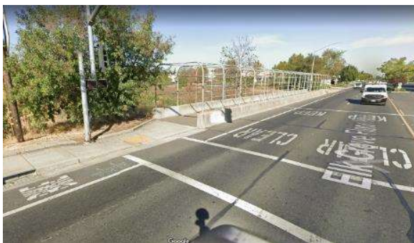
Figure 36. A photo taken from Google Maps Street View from 2020 showing the narrow space just outside of the caged sidewalk forcing bicyclists to make a sharp left turn to cross or wait for the pedestrian signal.
